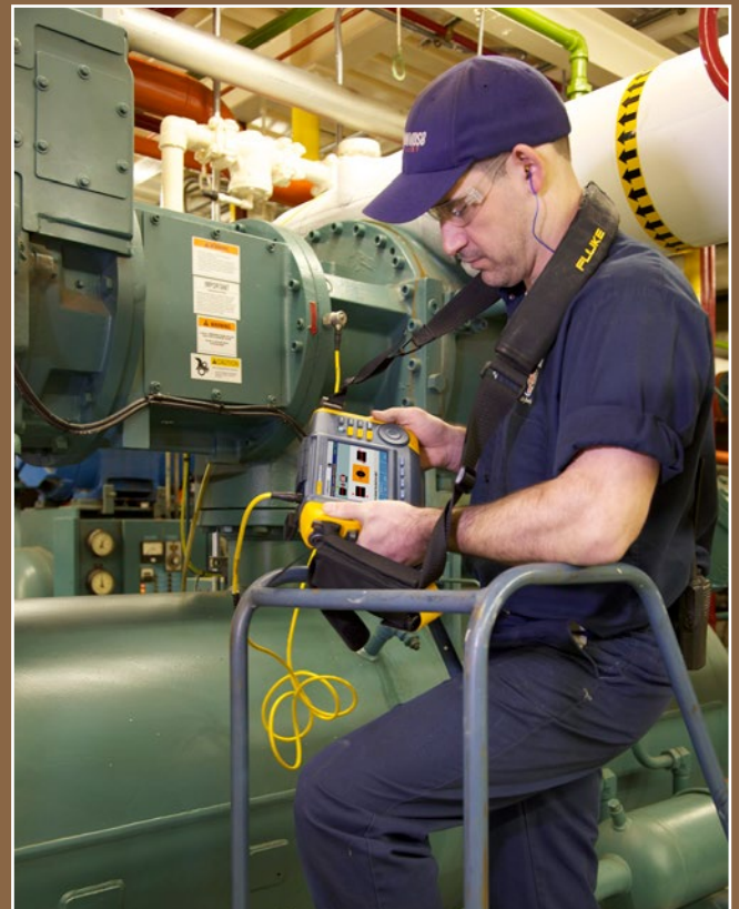
Figure 2: At Alpenrose Dairy, regular vibration analysis provides data for trend analysis used in proactive maintenance
