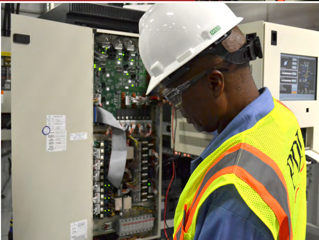
Figure 1: Field service technician verifies static transfer switch voltages and performs visual inspection during a routine PM visit
