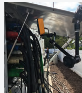
The thermal imager uses infrared technology to monitor a power cable located in the electrical panel of the Filmwerks' trailer
