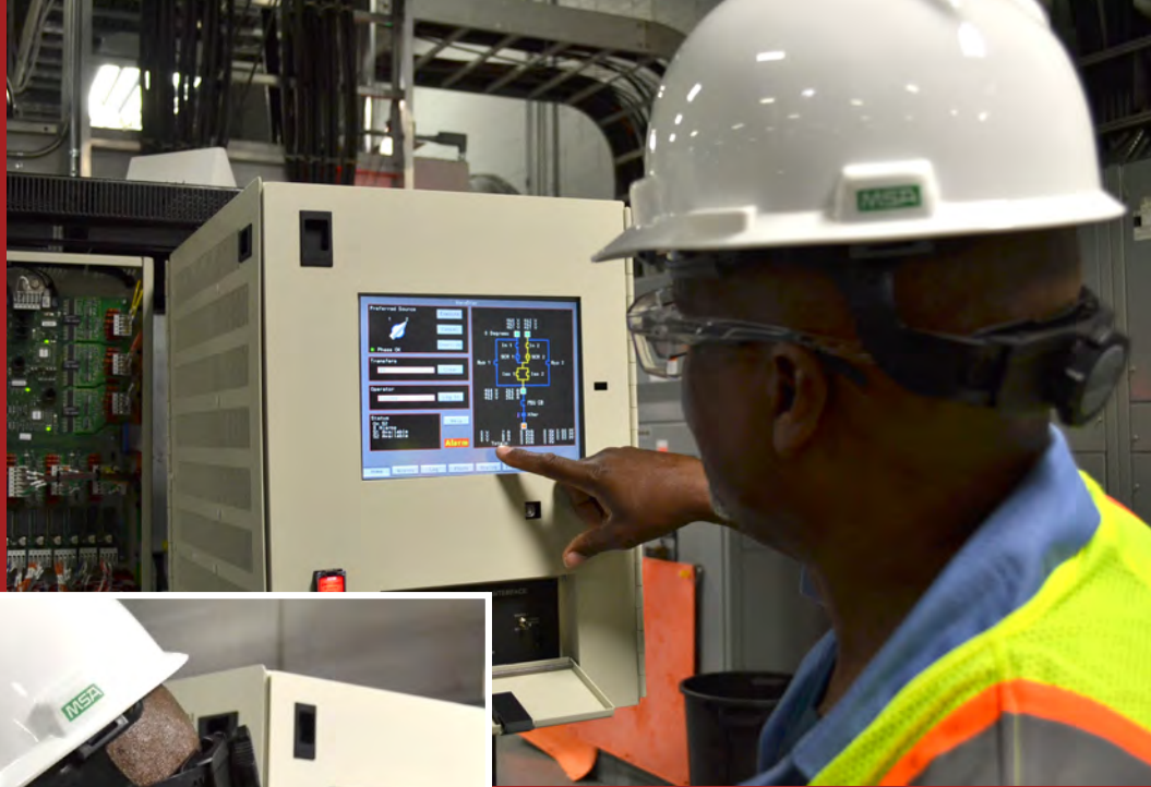
Figure 2: Field service technician confirming calibration and functionality on a static transfer switch during a routine PM visit
