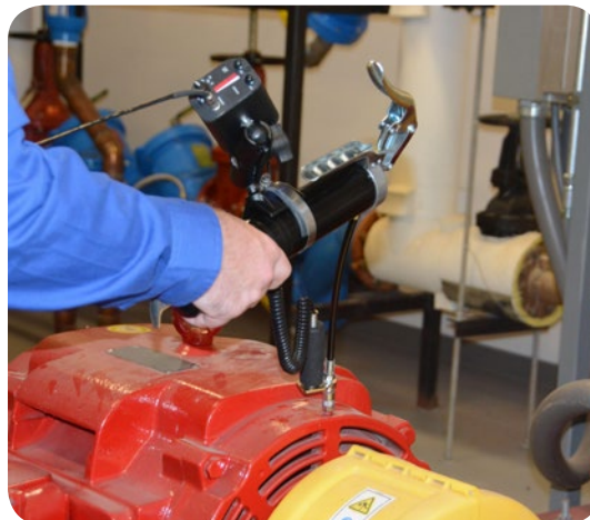
Figure 2: An ultrasonic lubrication delivery system being used (Photo courtesy of UE Systems)
