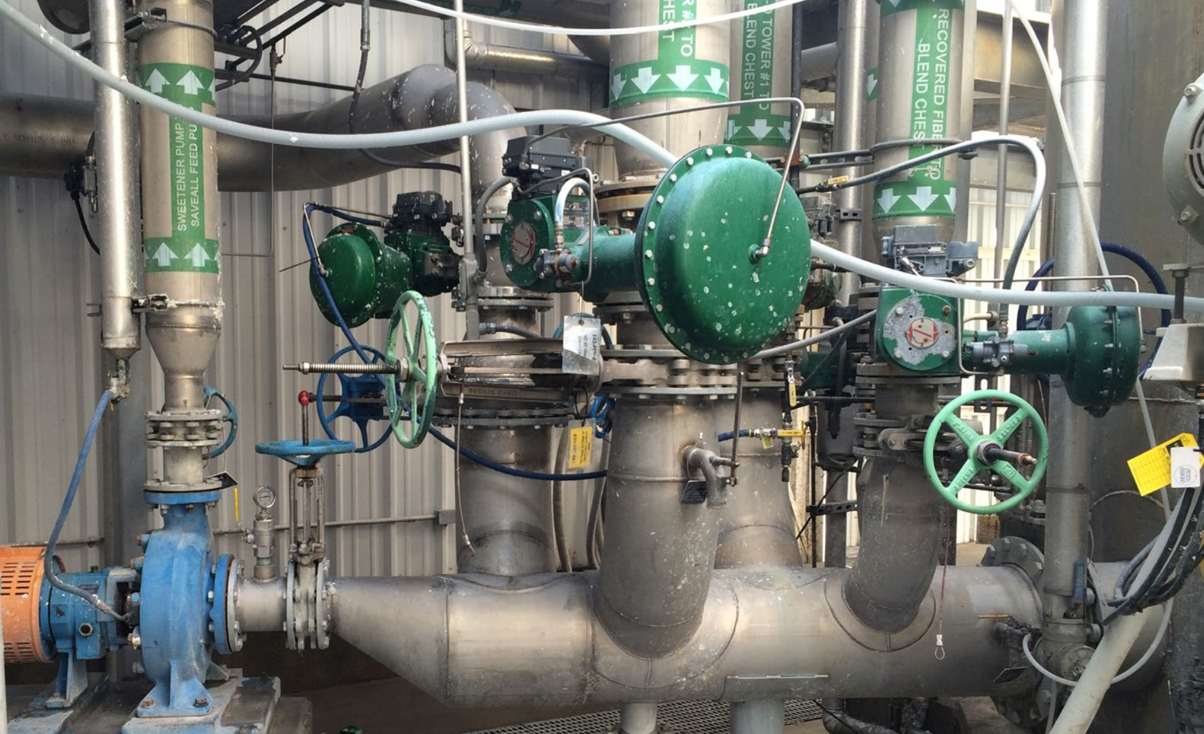
Figure 4: Design errors showing not enough straight run piping on pump suction
