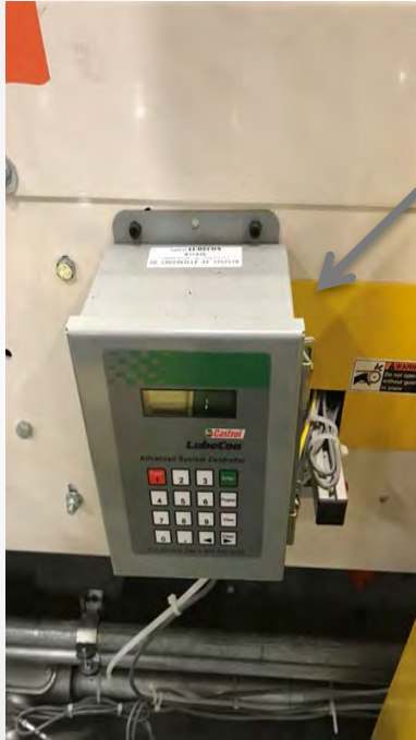
Automatic Chain Lubrication System
