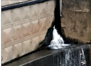
Closed lock gates with water leak in lower right-hand corner, Brandon Road Lock and Dam, Joliet, IL
